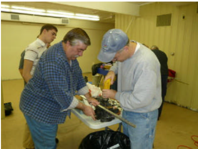
Fig 3. Drilling out our brackets. Larry K9LGP holds while Dave K9RUF drills. Mark KC9KCW (in the background behind Larry) offered many words of encouragement during this phase of the project.
