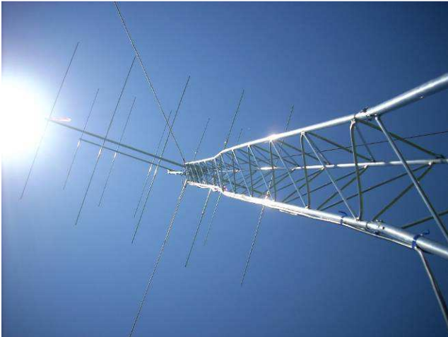
Fig 4. Looking up at the 6-Meter tower and array.
