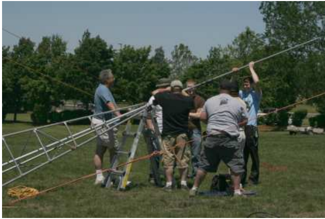
Fig 4. Getting the 6-meter antenna in the air.
